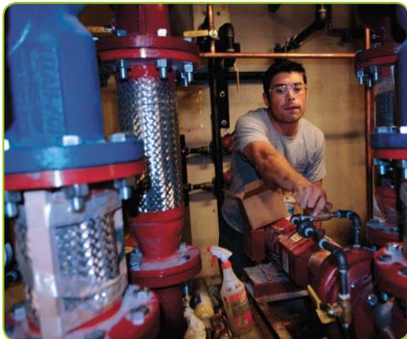
**Upgraded Boilers.** (554 Central, 899 Cleveland, 1085 Montreal and 325 Laurel (Neill)) The PHA upgraded hi-rise boilers to use more energy-efficient modulating-type burners and installed dual-fuel burners, to allow the PHA
